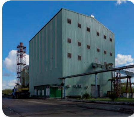
Since 2008, all bark waste along with sewage treatment plant sediments have been burned to produce thermal energy in a large-capacity waste-heat boiler, and the ash generated by waste incineration is cooled and disposed in an environment-friendly manner.
